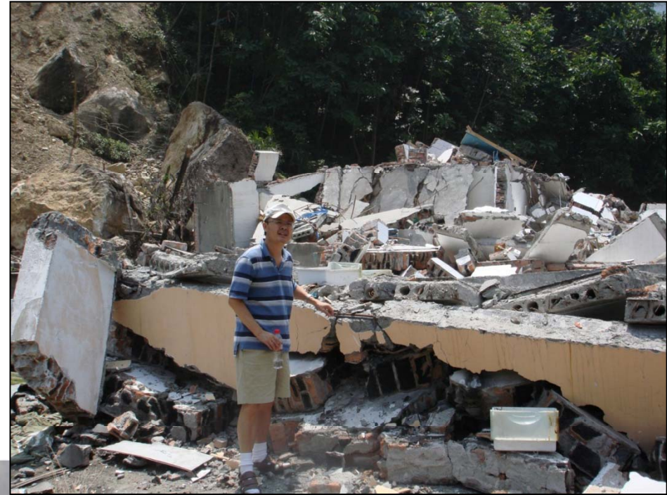
landslide crushed some buildings in Beichuan.
