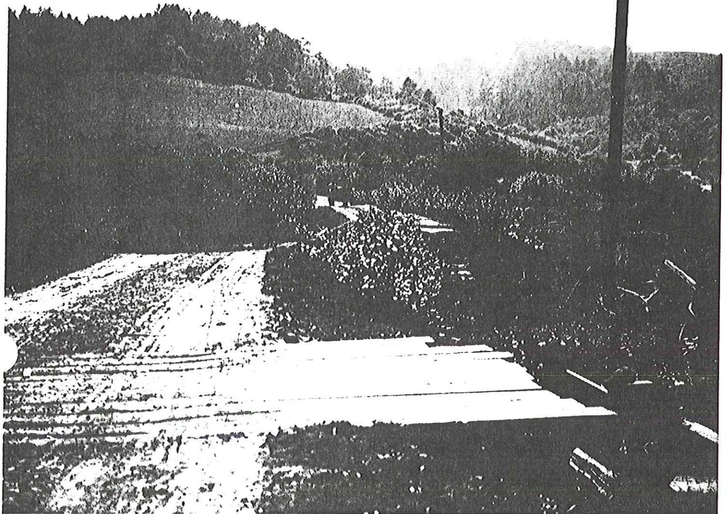
Figure 6.4 Right-lateral horizontal movement of the San Andreas fault in the 1906 earthquake across the old Sir Francis Drake Highway north of San Francisco, at the southern end of Tomales Bay, California. The offset was 6.5 meters (20 feet). [Photo by G. K. Gilbert; courtesy of USGS.]
